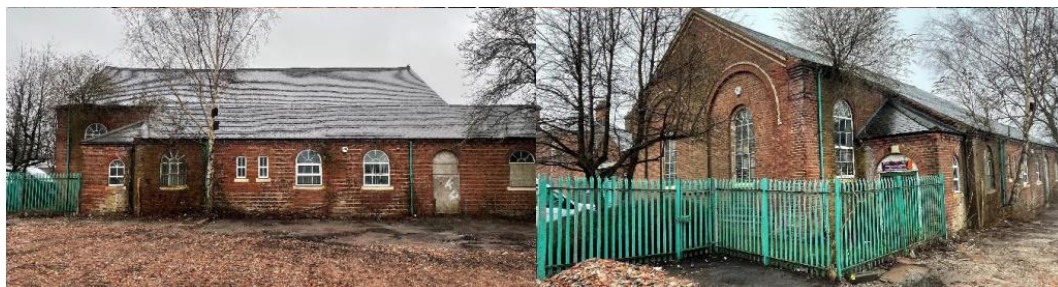
Figure 14: Current photos taken of Building A
